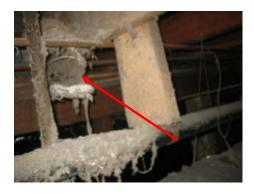
FYI: A cover plate is noted missing at the receptacle in the Laundry Room
