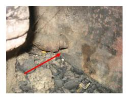
The gas valve at the fireplace cannot be turned due to the presence of debris (SEE PHOTO). Recommend clearing debris from exterior of gas valve to allow for proper operation.
