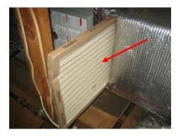
FYI: The filter size for both HVAC units is 16" x 25" x 1." The filters should be replaced at least once every three months.
