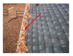
A small area of wood rot is noted at the fascia board on the west side of the covered deck (SEE PHOTO). Recommend repair or replacement of damaged wood.
